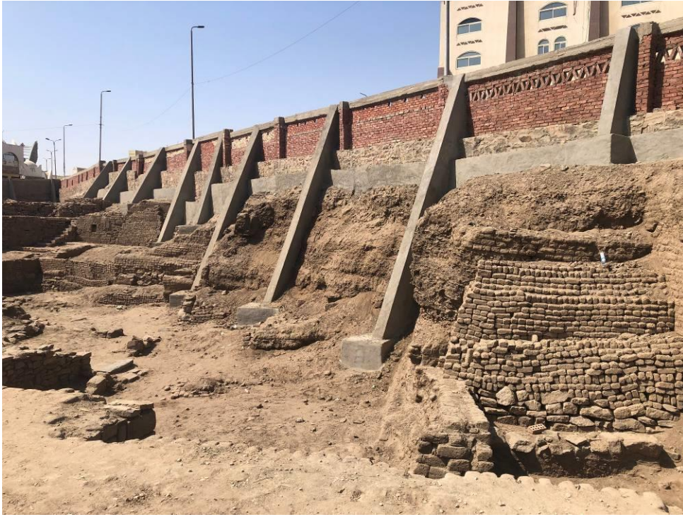
Fig. 49: Area:2: View of the reinforcement of the western perimeter wall (southern part).
